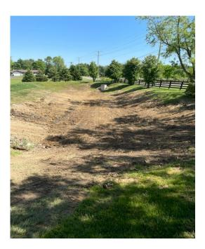
Before and after pictures of a dry basin where the cattails took over and clogged the underdrain in the basin. Ditch maintenance staff removed all cattails, replaced the underdrain and installed a surface inlet. The basin was then finish graded and seeded.
